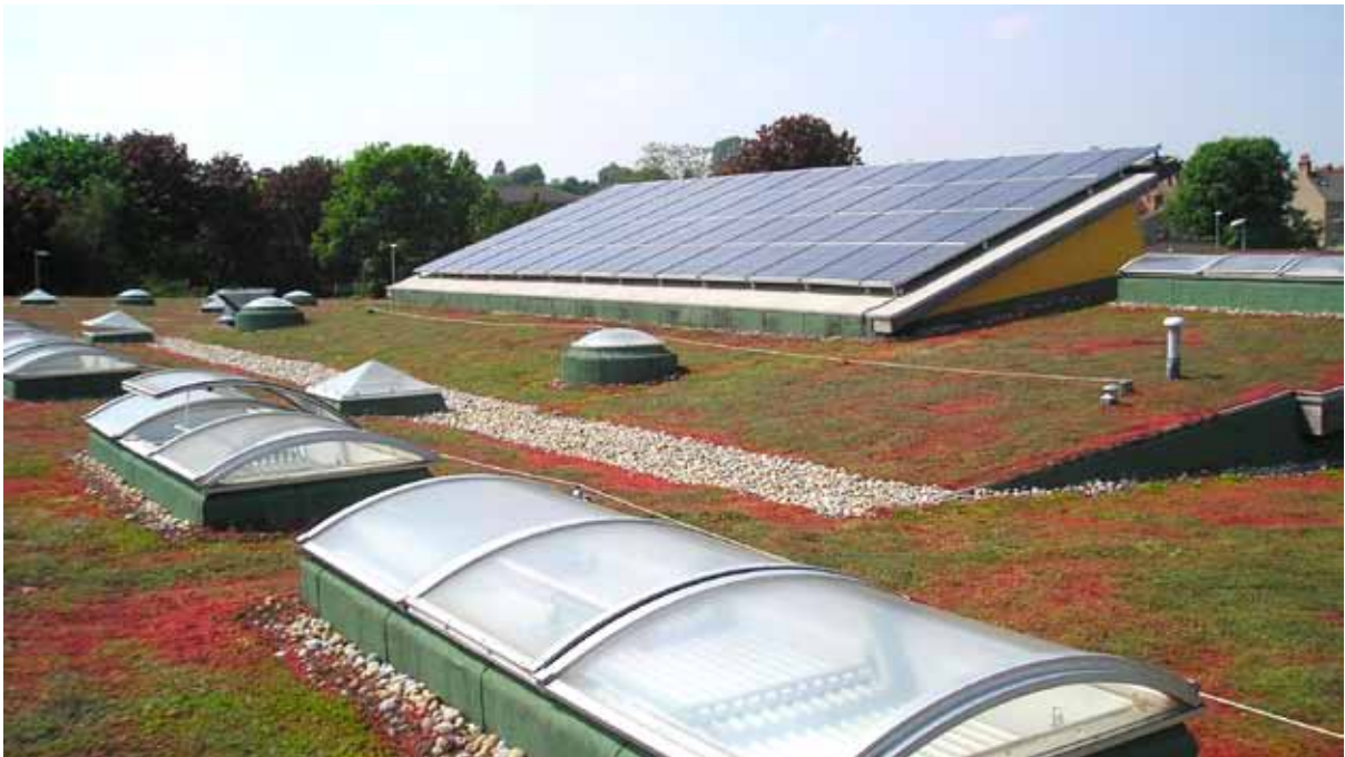
Green roof, photovoltaics and sun lights at Orchard Primary School, Sidcup
