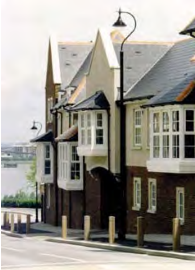
Ingress Park, Greenhithe, Kent
