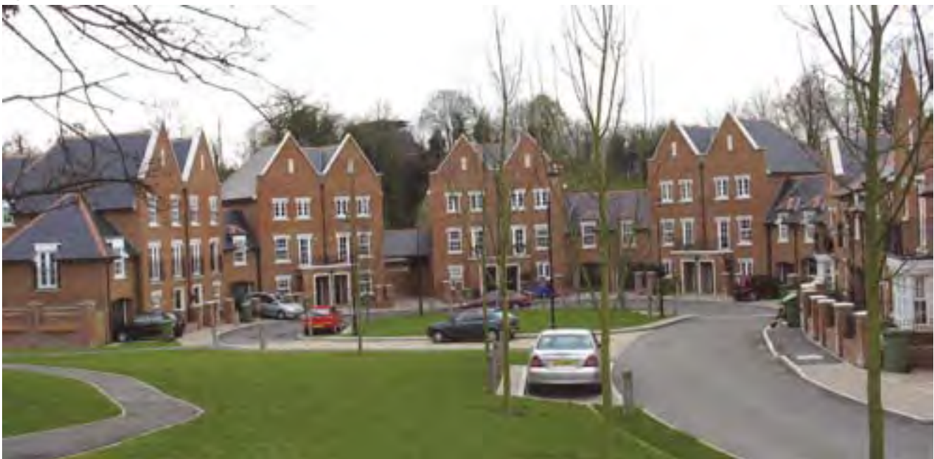
Ingress Park, Greenhithe, Kent
