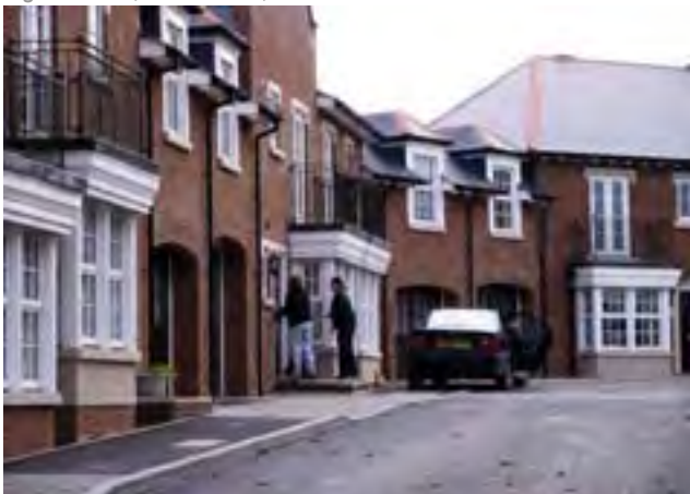
Ingress Park, Greenhithe, Kent
