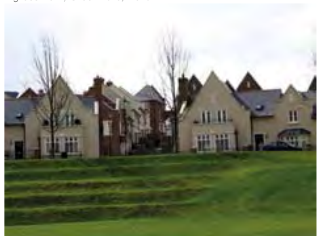
Ingress Park, Greenhithe, Kent
