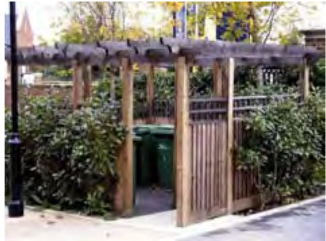
Ingress Park, Greenhithe, Kent
