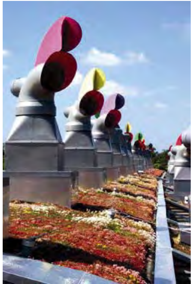
This roof incorporates a permeable surface to reduce surface water run-off and wind ventilation shafts.
