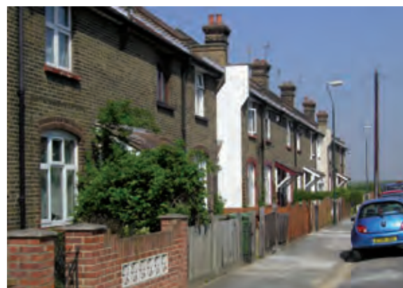
Oak Road, looking east, which shows the uniform pattern of groups of terraces
