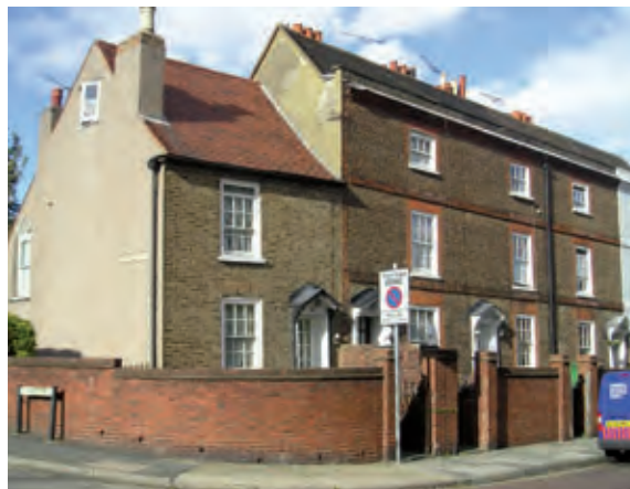
64-56 Bexley Lane (Grade ii Listed)
