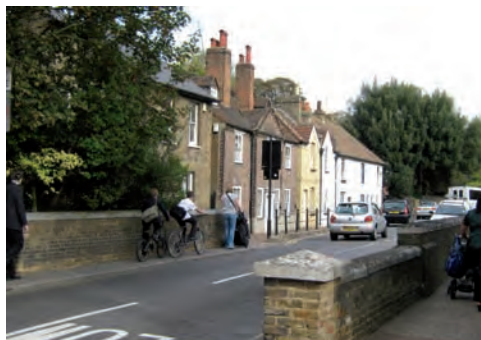
Road bridge over the River Cray
