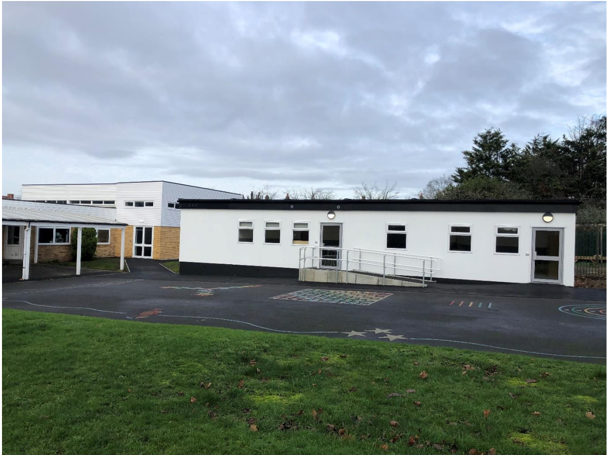
Image of Aspire SEMH Expansion completed in November 2020.
