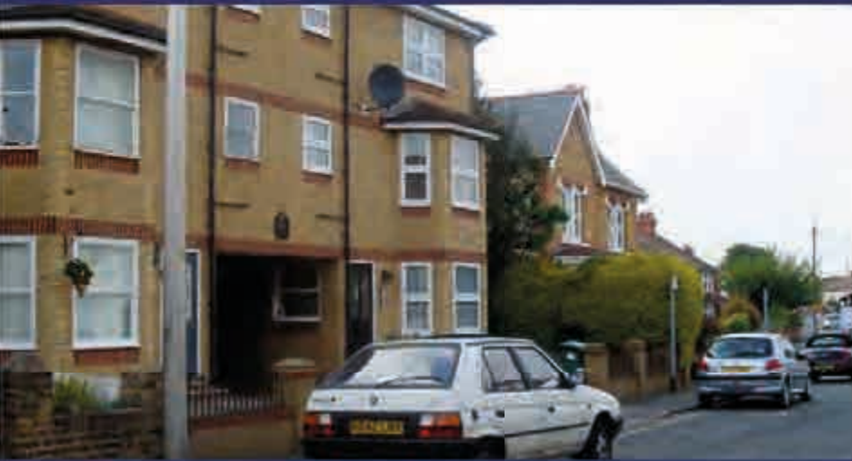
←←← Examples of the residential areas that surround the town centre.
