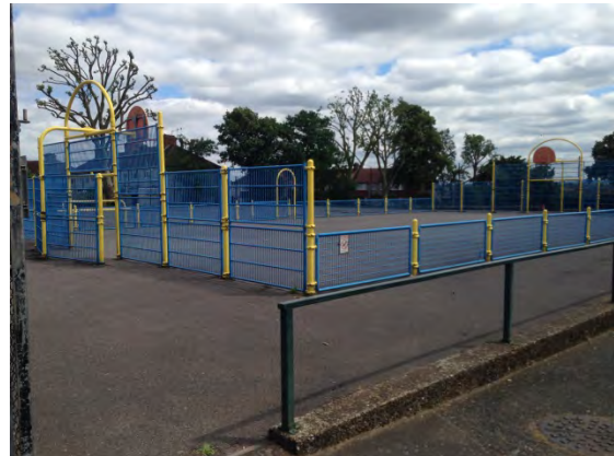
MUGA at West Heath Recreation Ground.
