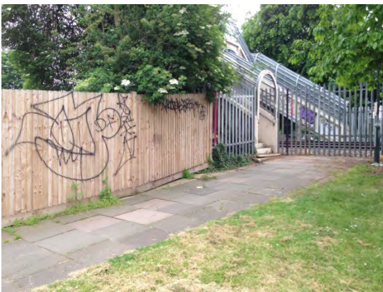
Evidence of graffiti at Old Farm Park (West).
