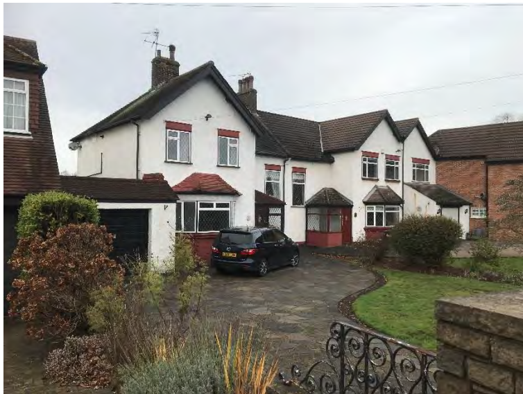
Photo 3: View of 6-8 Danson Road looking northwest
