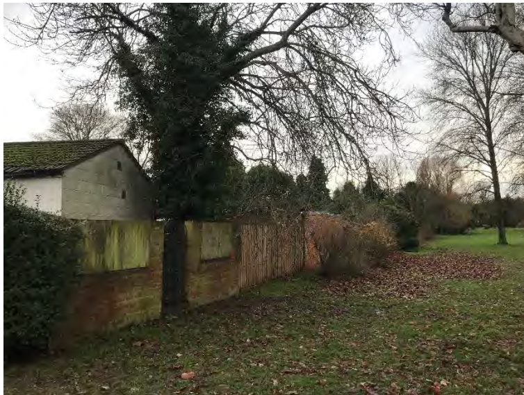
Photo 5: View of the rear of the Site looking south from the northwest corner
