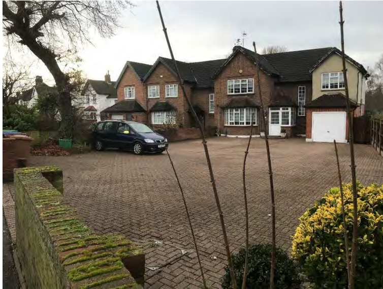
Photo 4: View of the Site looking southwest
