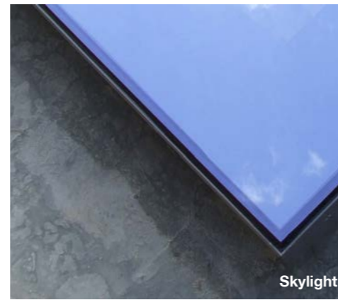
Polyester powder coated aluminium frame
