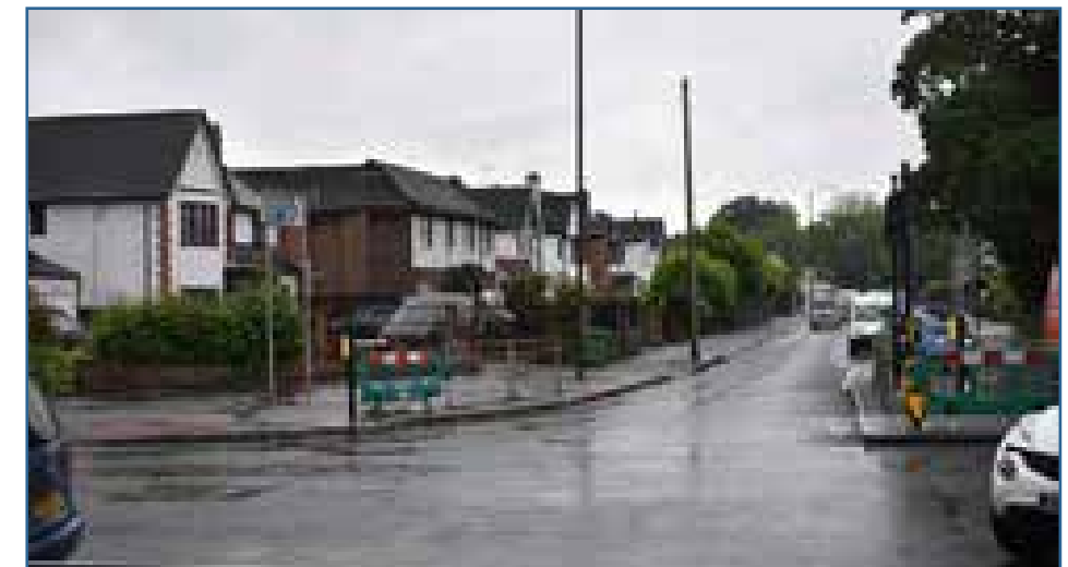
View of characteristic, linear 2 storey development along Danson Road.
