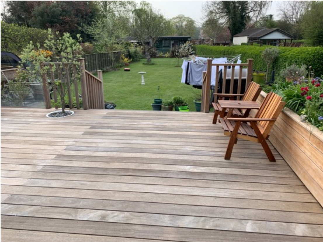
Photograph 7: Rear garden of 6 Danson Road, looking west
