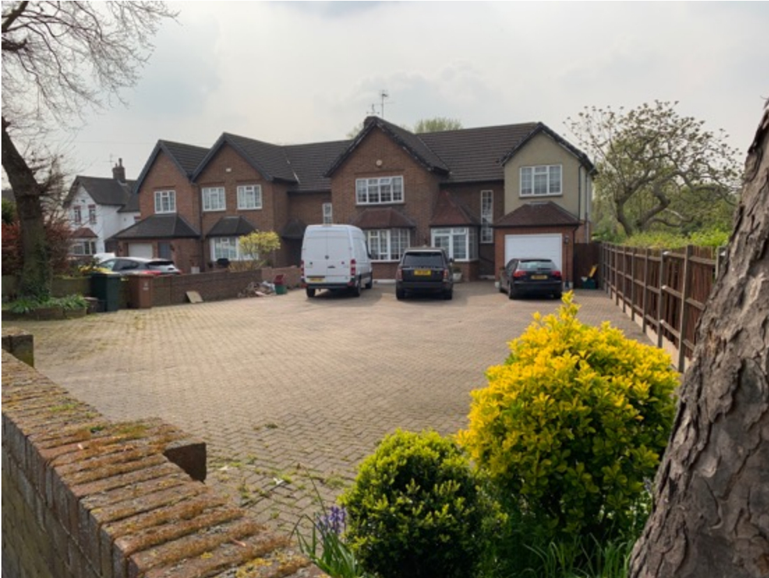
Photograph 1: Front of 2 and 4 Danson Road, looking south-west
