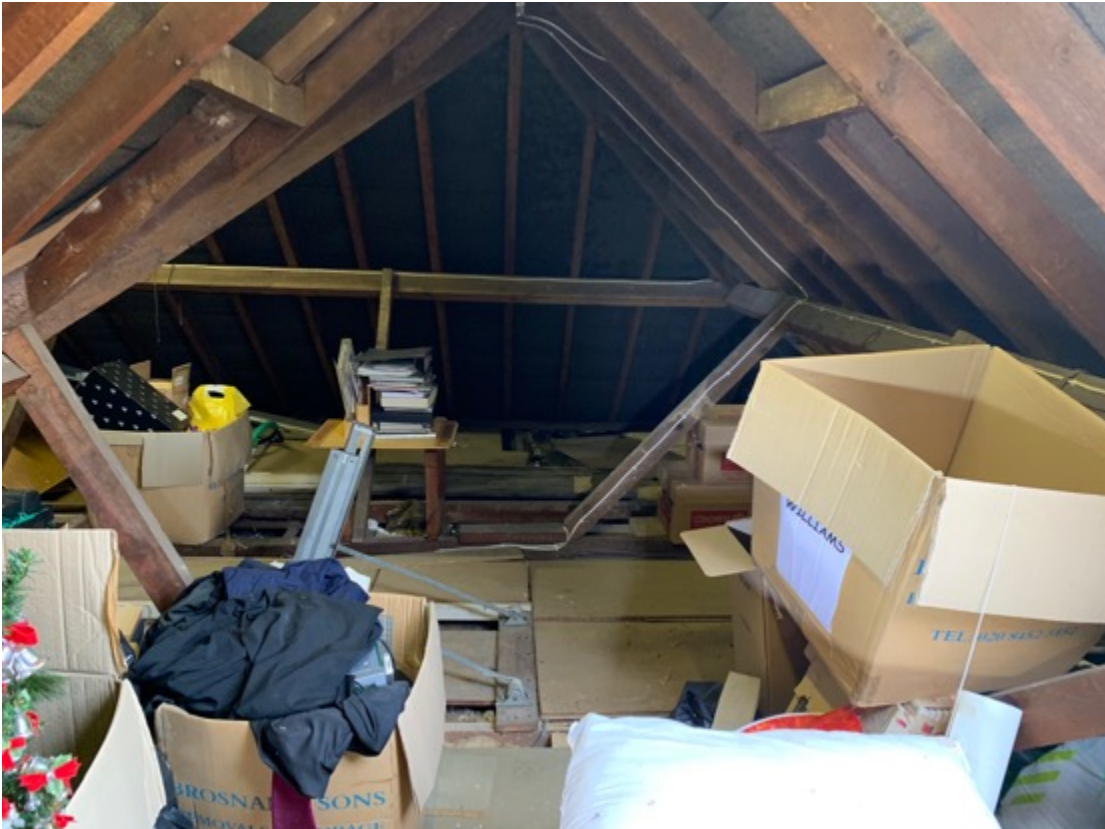
Photograph 11: Internal roof void of 6 Danson Road (no evidence of bats)
