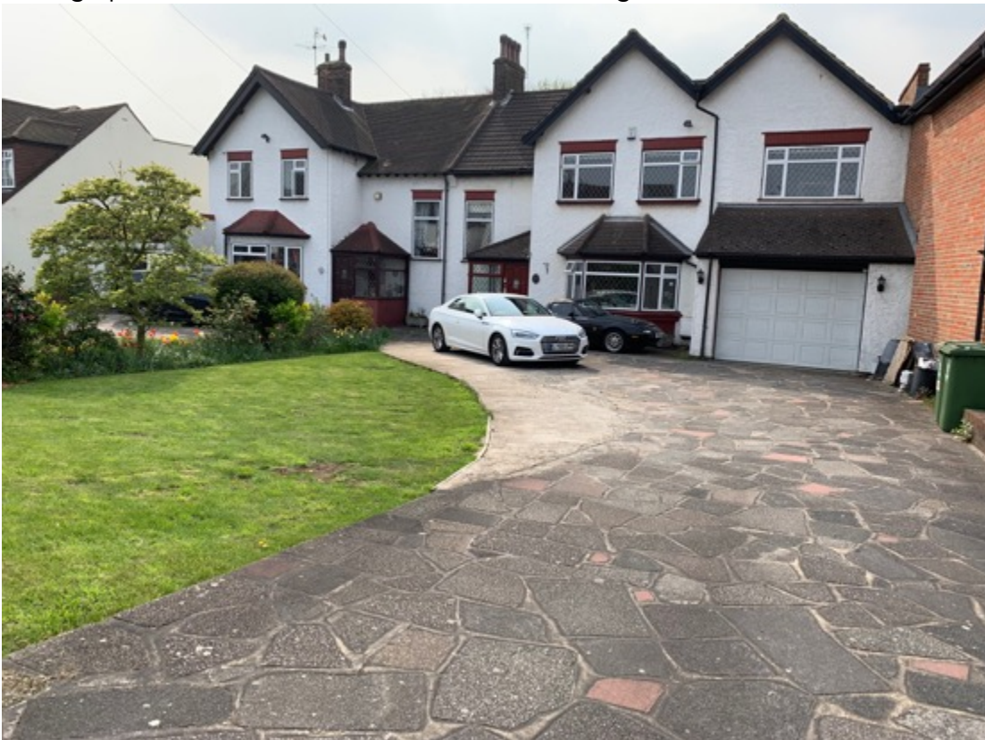
Photograph 2: Front of 6 and 8 Danson Road, looking south-west
