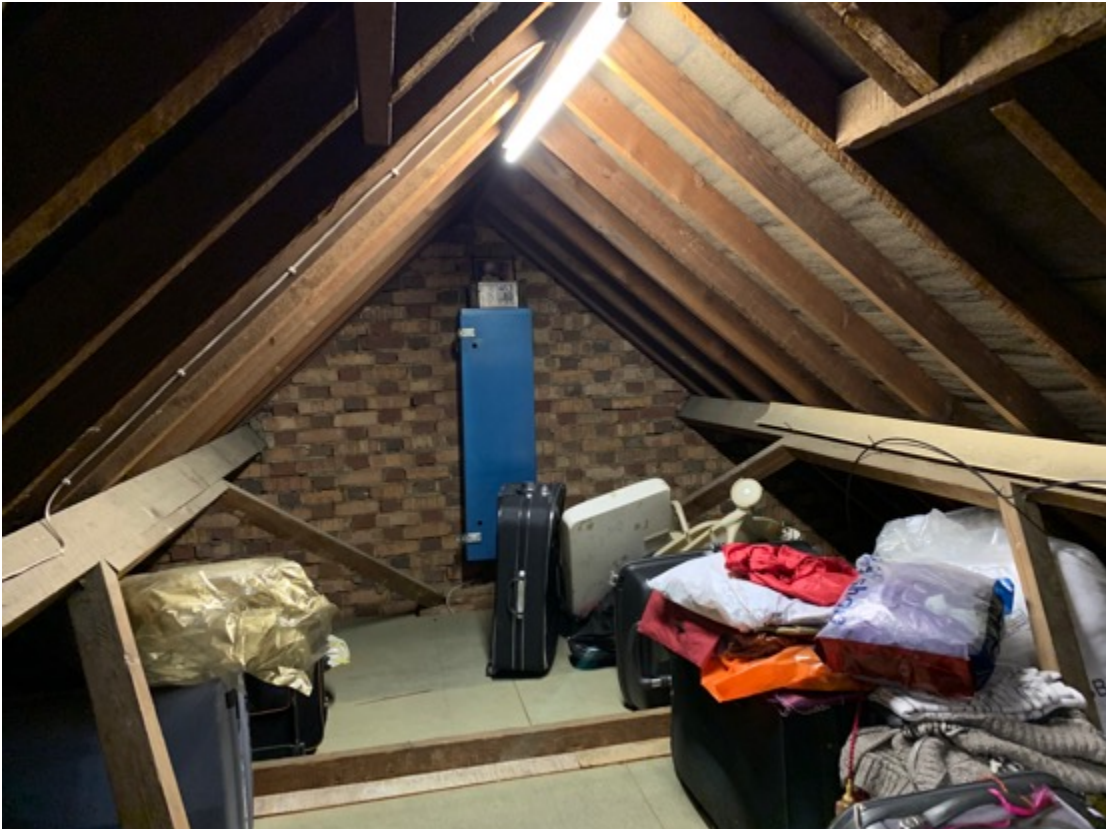
Photograph 9: Internal roof void of 2 Danson Road (no evidence of bats)
