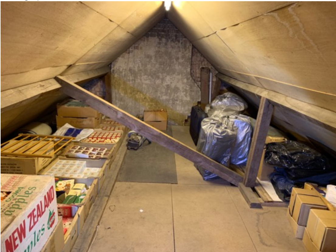
Photograph 12: Internal roof void of 8 Danson Road (no evidence of bats)
