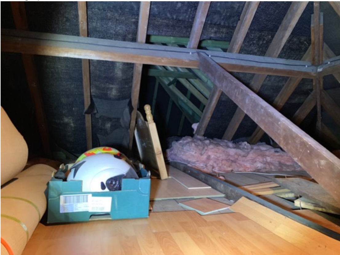
Photograph 10: Internal roof void of 4 Danson Road (no evidence of bats)
