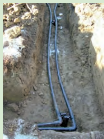
Ground works for ground source heating
