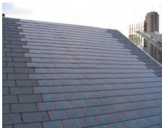
Above: Solar thermal tiles
