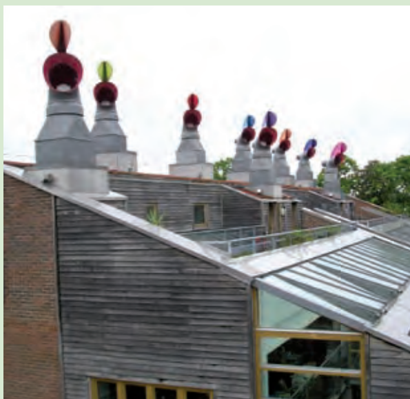
Passive stack ventilation, BedZED development of homes, community facilities and workspace at Wallington, South London
